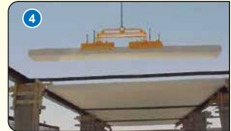
Install the slab adjacent to each other.
