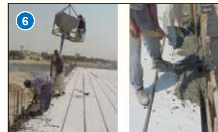
Make a circular rib from the outside of the slabs to tie them
