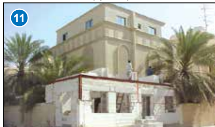
The building upon installing the slabs
