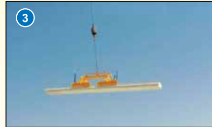
Lifting the slabs to be installed
