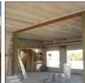
Span over 6 meter
