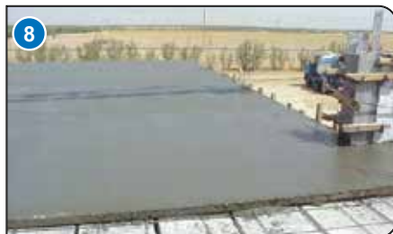
Cast a concrete layer of maximum 7 cm thickness (optional).
