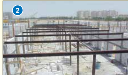
Iron skeleton before installation in wide buildings
