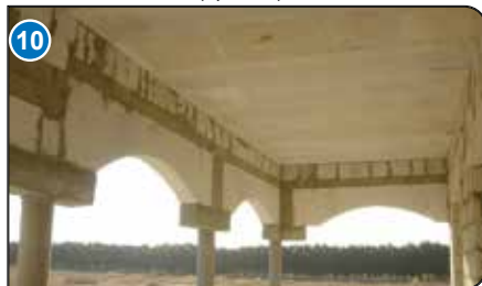
The look of slabs after installation.
